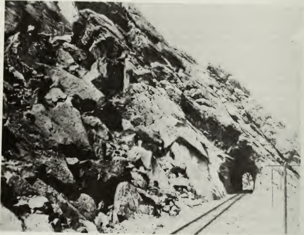
The Moffat Road, along Coal Creek Canyon, was a feat of engineering as this 1909 photo shows. M. R. Campbell Photo, Courtesy USGS
